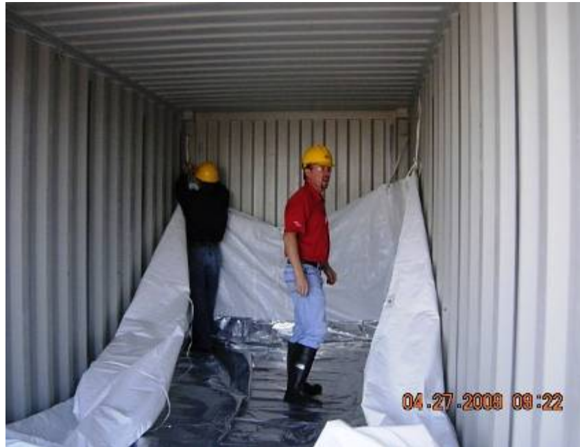
Photo #1 Barrier Wear Sleeve Liner Installation
