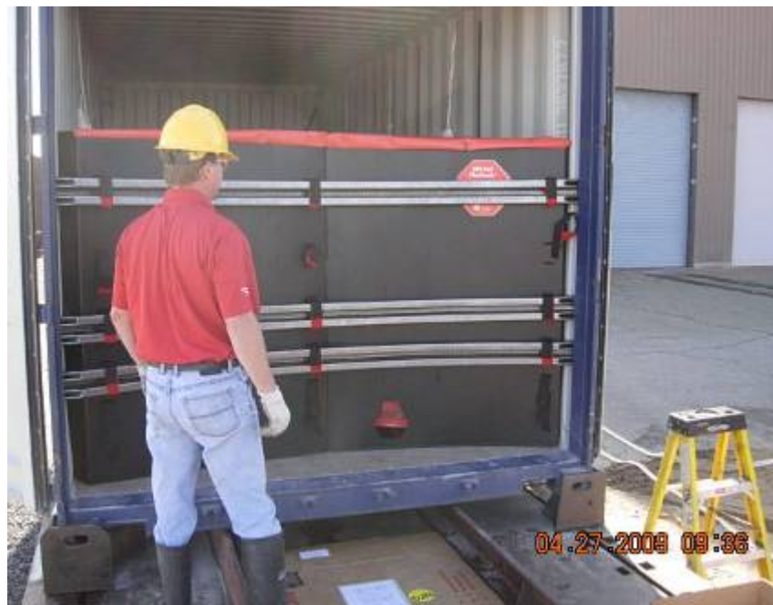
Photo #4 Bulkhead Installation
