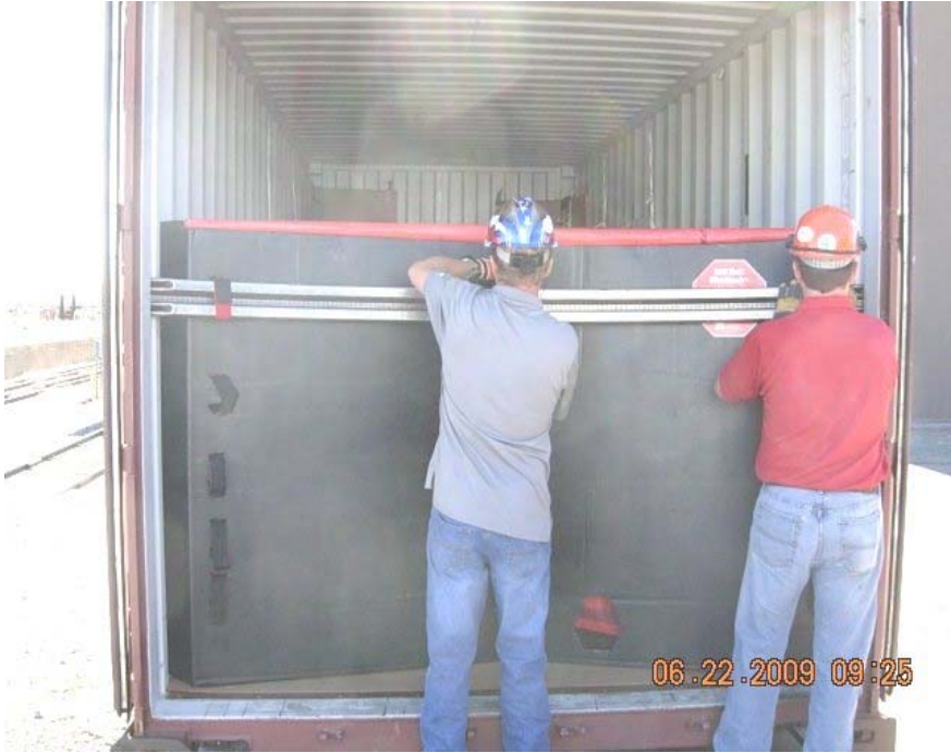
Photo #3 Bulkhead Installation
